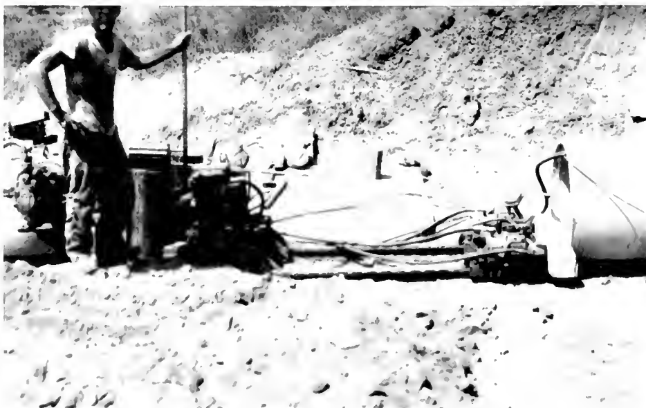
Excavated material about to be removed
